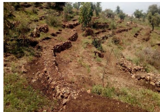
Figure 4: Anti - erosion measures in progress
