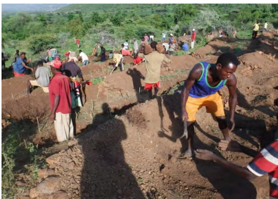
Figure 3: Community terrain works on the slopes
